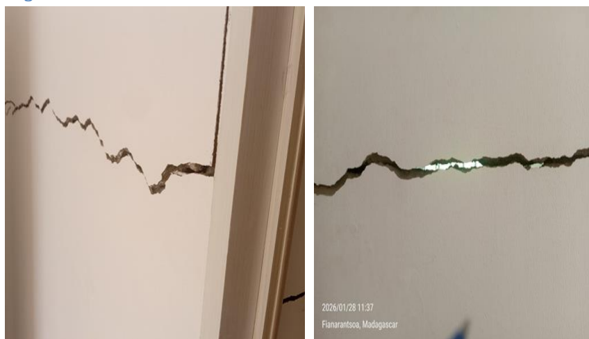
Figure 4: MCC de Haute Matsiatra
