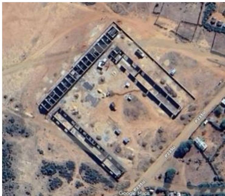
GYMNASE DE 1000 PLACES AMPANIHY
